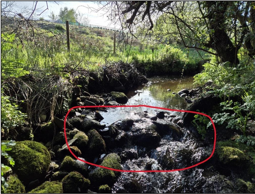
Figure 2-3 - Natural rock to be sealed with small sandbags for Dam 2 located downstream of Carrowrevagh Bridge
